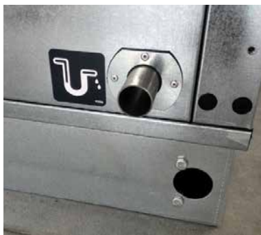
Condensate drain for plate recuperation
